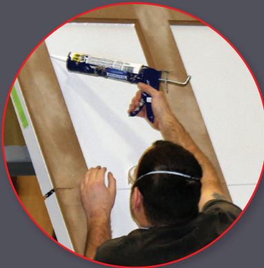
Overlay is permanently adhered to door sections, all joints are sealed with weatherproof caulking/sealant
